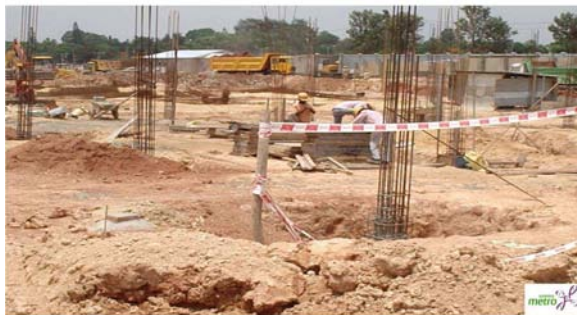
REINFORCEMENT WORK IN PROGRESS
