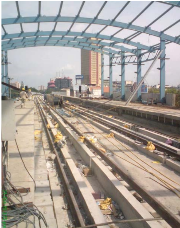
Track and system works in progress at MG Road Station
