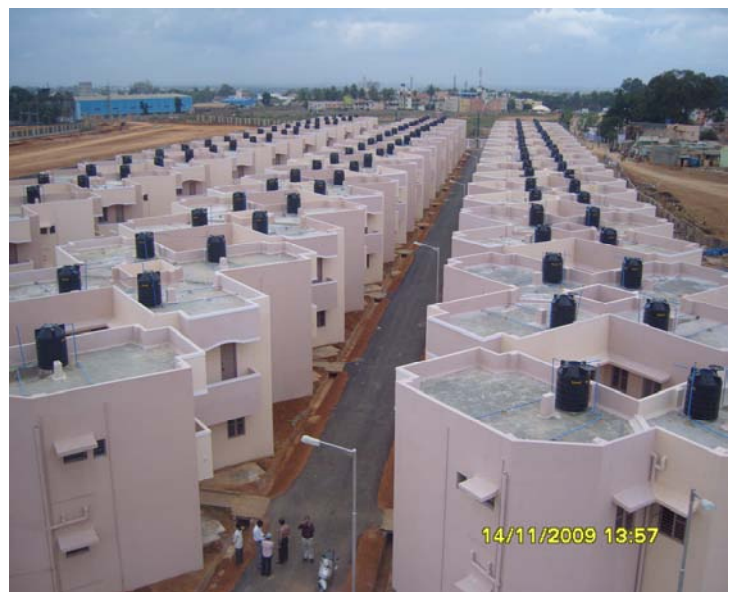
Peenya Rehabilitation Row houses
