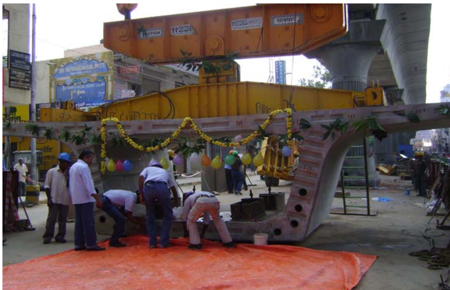
Last Segment of Reach-1 was launched on 1st September, 2010
