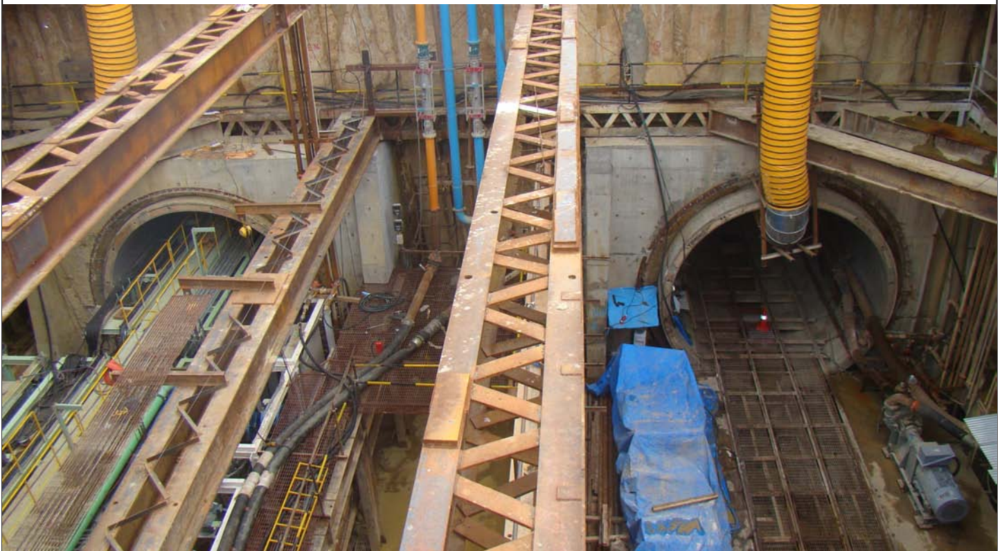
Twin Tunnel Work in Progress.
