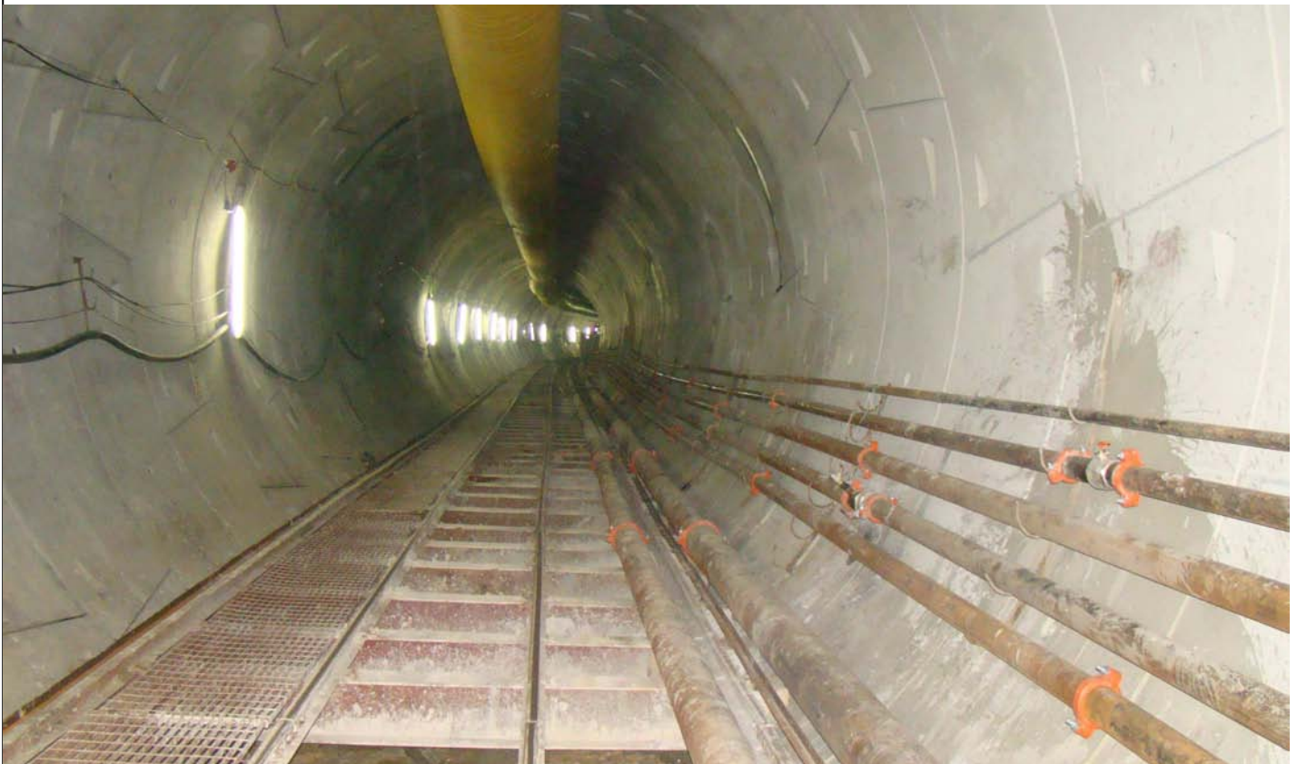
Tunnel view of UG corridor by TBM
